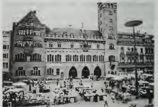
The Rathaus (town hall), Basel, Switz., fronted by market stalls
